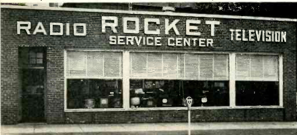
Rocket Stores found it necessary to build this separate Service Center. Servicing business then expanded four times. Manufacturers use it as a base for field trips and to test new TV receivers.
